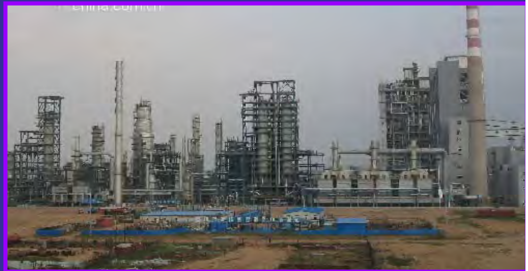
Shenhua's coal-to-liquids plant in Ordos
