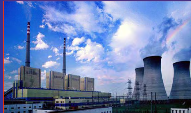
Gaobeidian power plant in Beijing
